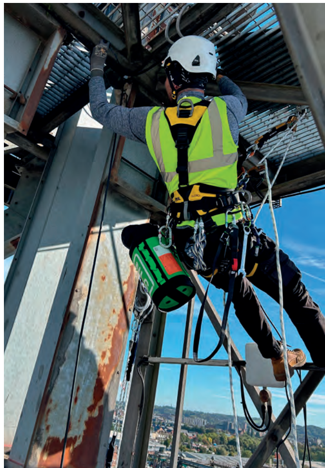
Skilful installation of IE node electronic monitoring equipment on a silo elevator at Shobnall Maltings, Soufflet Malt, Burton on Trent, England.
