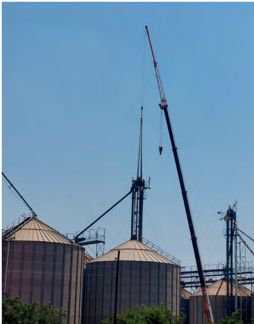
Elevator buckets being fitted on an 85 meter belt at Schoeman, Boerdery, Delmas, South Africa.
