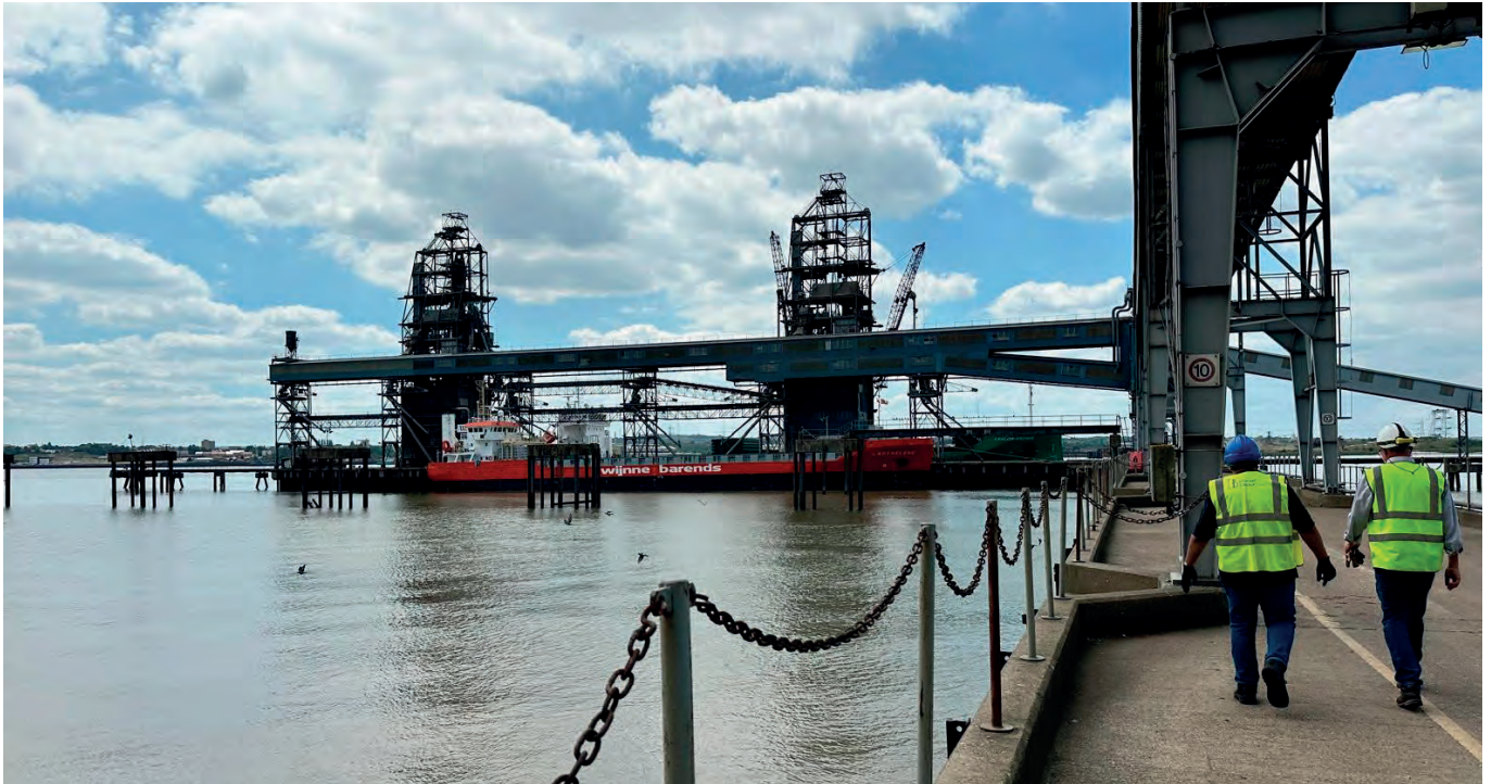
Loading and unloading berths at Tilbury Docks utilising 4B Group engineering components.
